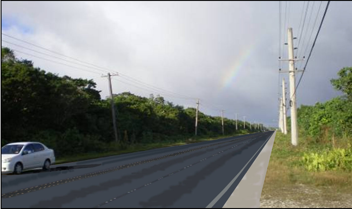
Figure 13.2-18. Alternative 8: View from Route 3 Looking Northward into the North Part of NCTS with New Facilities in the Foreground (RESULTING VIEW)
