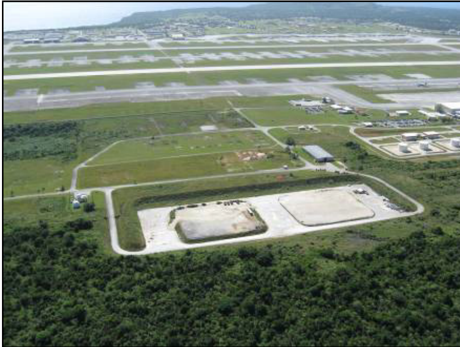
Figure 13.1-2. Aerial View of the North Ramp Area looking from the Northeast to the Southwest with Heavily Vegetated Cliff line in the Foreground
