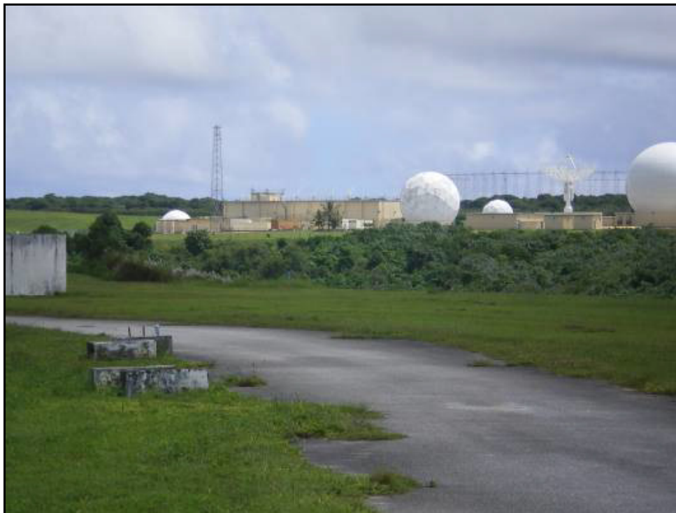
Figure 13.1-13. NCTS Finegayan Communications Facilities
