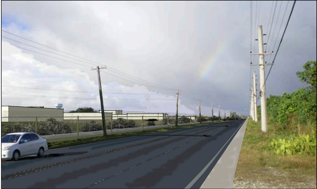
Figure 13.2-10. Alternative 2: View from Route 3 Looking Northward into the North Part of NCTS with New Facilities in the Foreground and Water Tower/Tank in the Background (RESULTING VIEW)
