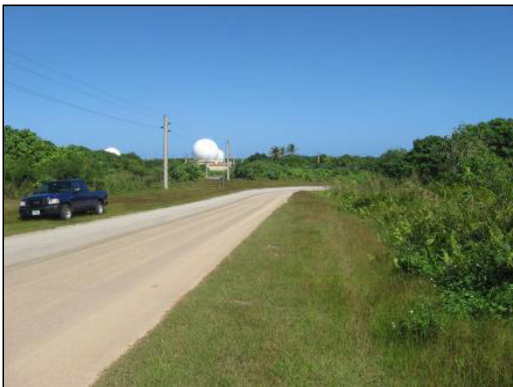
Figure 13.1-11. A Typical View from Within the NWF Area
