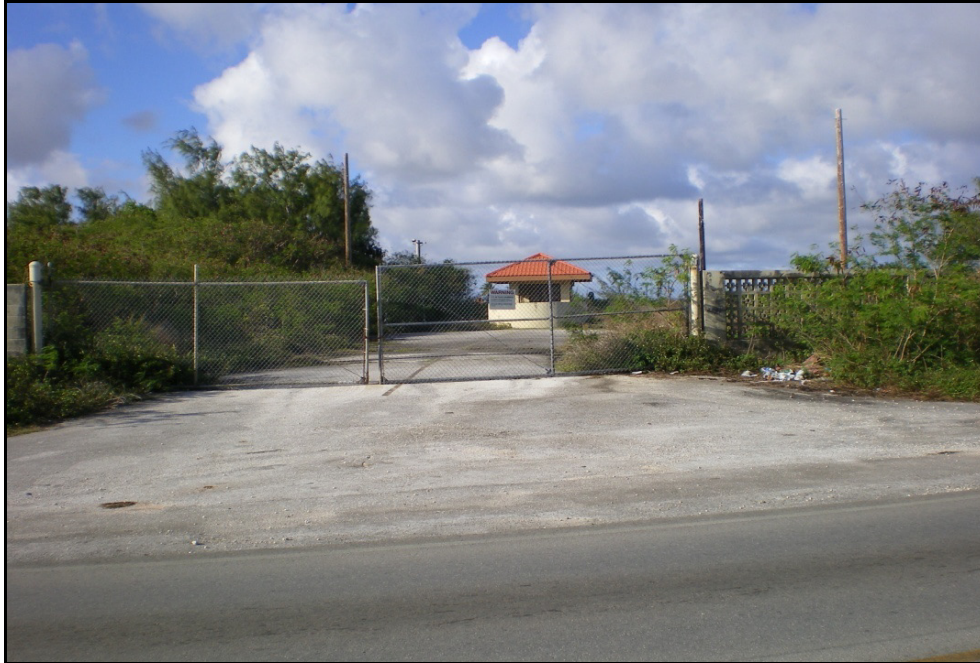
Figure 13.1-29. View of Andersen South Gate from Route 15 Source: EDAW 2008.
