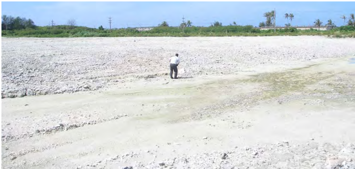
Figure 10. Existing Conditions in 2007 at Field 5 Dewatering Facility, Cell 1, between Sumay and Marina Drives, Apra Harbor, Guam
