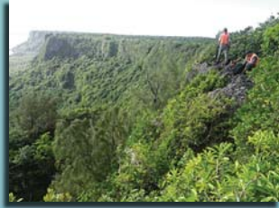
Clifflines provide a natural barrier
