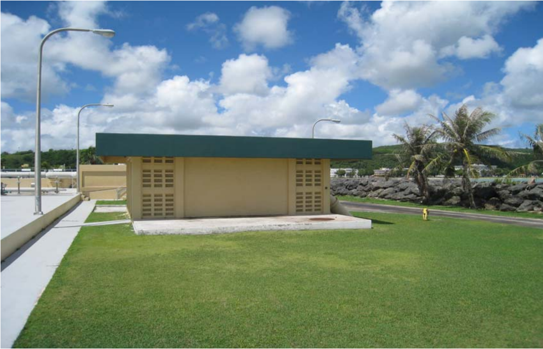
Effluent Pump Station
