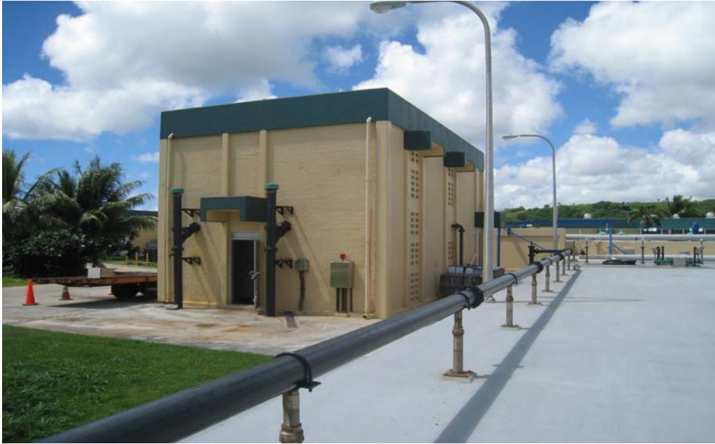
Sludge Dewatering Building
