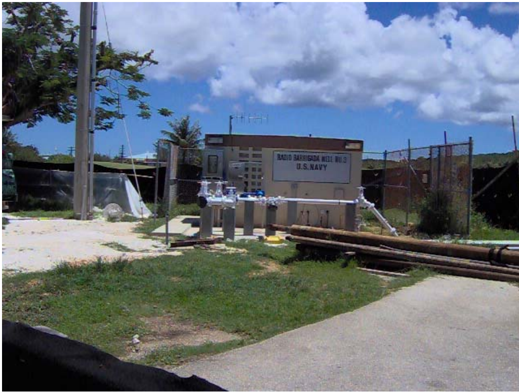
Rehabilitation at NCS 3 – June 09
