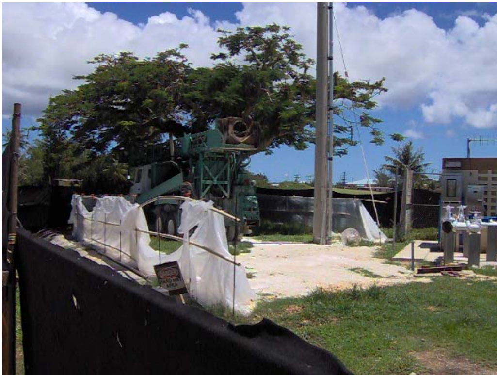
Rehabilitation at NCS 3 – June 09
