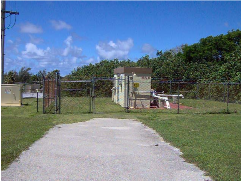
Rehabilitation at NCS 8 – June 09
