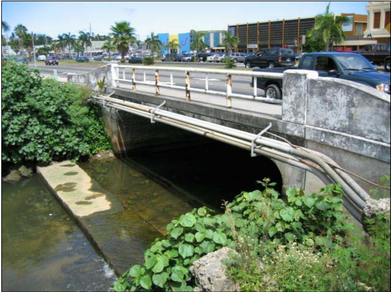
Contemporary View of Agana Bridge #1 showing parapet walls and railings
