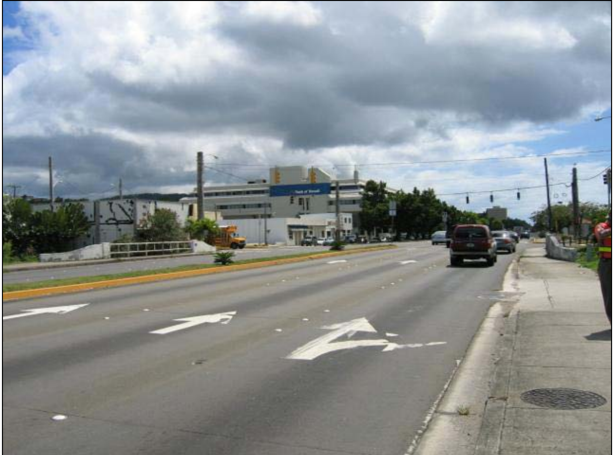
Contemporary View of Agana Bridge #1 and Route 1
