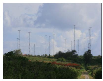
Figure 12.1-4. Antenna Array of Mariana Relay Station
