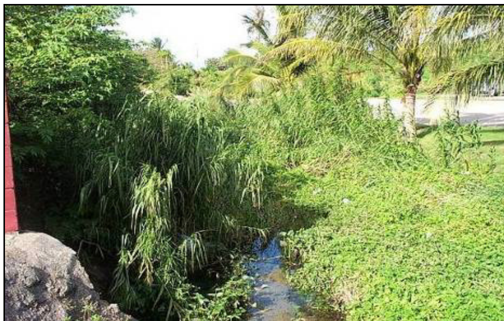
Figure 4.1-18. Tamuning Drainageway Downstream Channel
