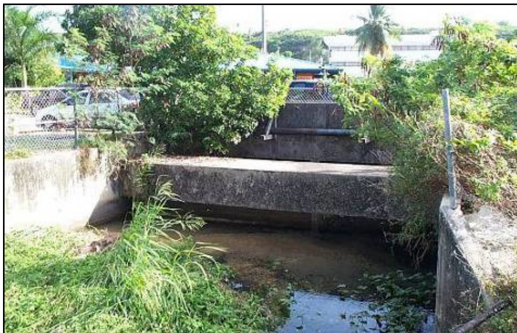
Figure 4.1-17. Tamuning Drainageway Outlet
