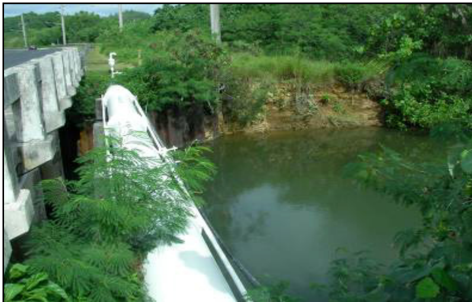
Figure 4.1-34. Route 1 at Atantano Bridge
