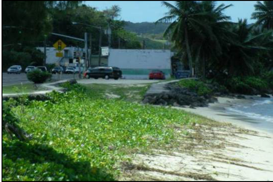
Figure 4.1-27. Coastal Erosion Protection along Route 1
