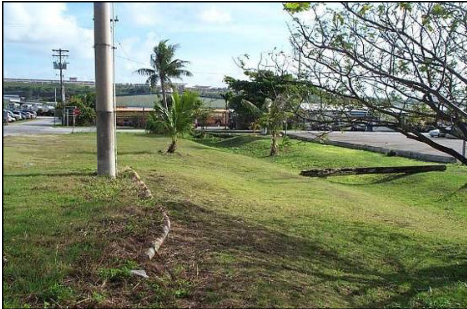
Figure 4.1-10. Grass Swale along Route 1 in North Area
